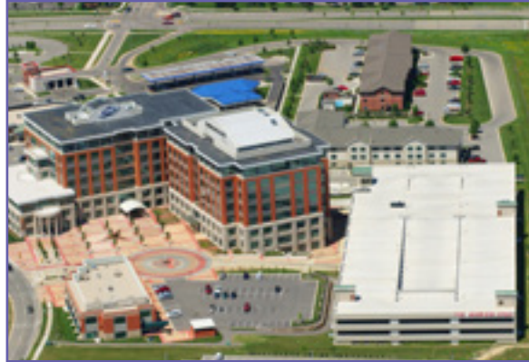
Parking Options / Surface and Ramp
