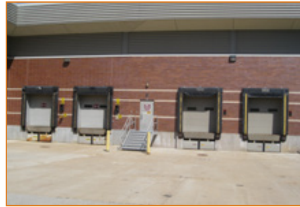
Loading Docks & Drive-In Doors at 726 Heartland Trail
